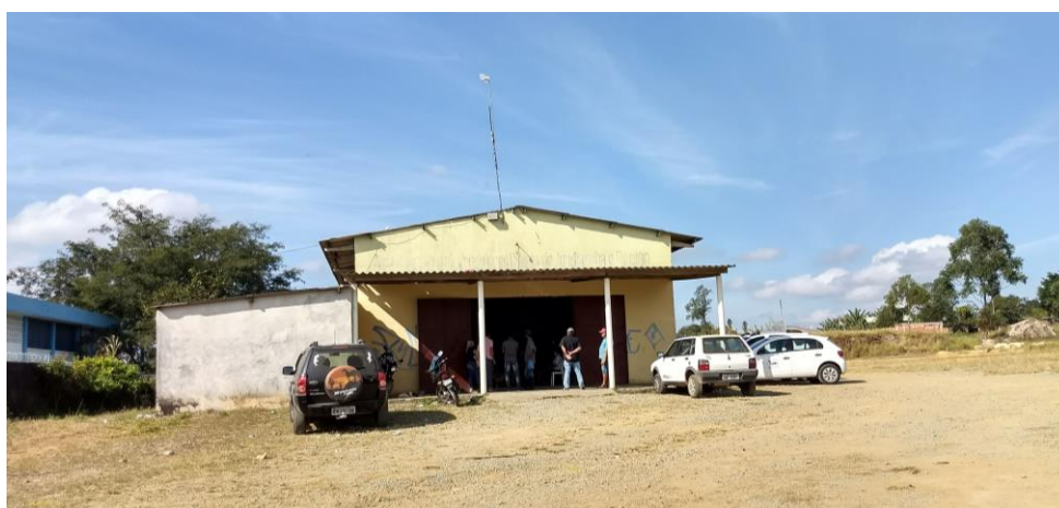
Figure 1 Current distribution point. Source: Authors
